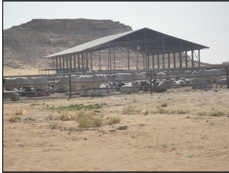
Figure 3: Part of quarantine facility at Wadi Halfa, 2012
